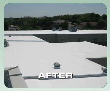
Apply highly reflective finish coat to roof at recommended rate. Start saving energy immediately.
