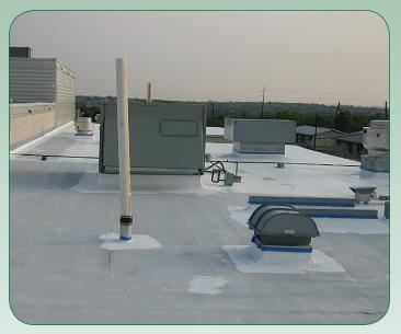
Apply basecoat at recommended rate. Backroll any vertical surfaces (parapets, walls, etc.).
