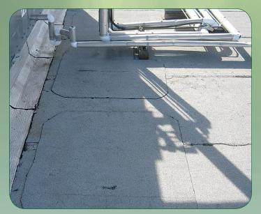
Repair and replace any deteriorated areas with **LIKE MATERIALS** to make **WATERTIGHT**.
