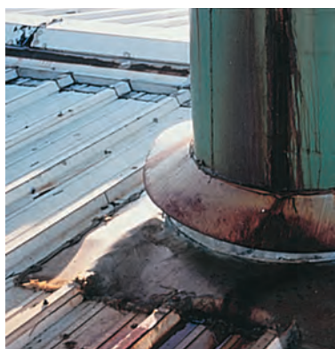
Cracks or leaks around penetrations.
