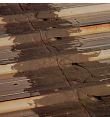
Seam and fastener problems.
